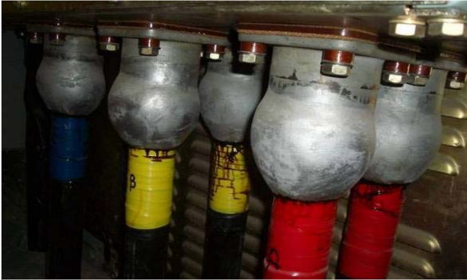
Solidly bonded - lead plumbed
