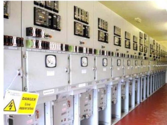
Switchgear (Air, Solid, Gas-insulated)
