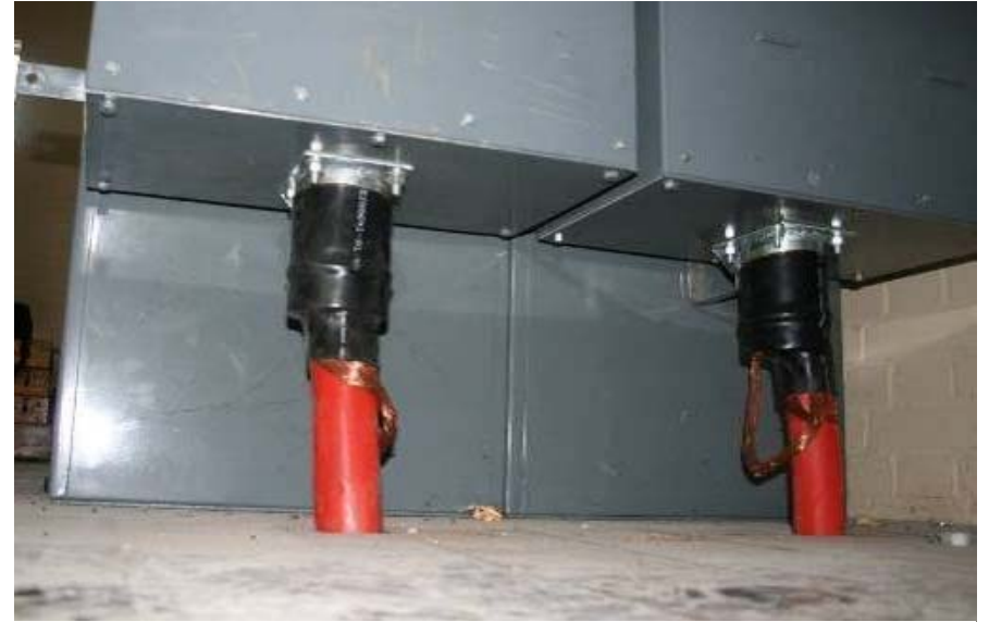
Solidly bonded - No insulated gland
