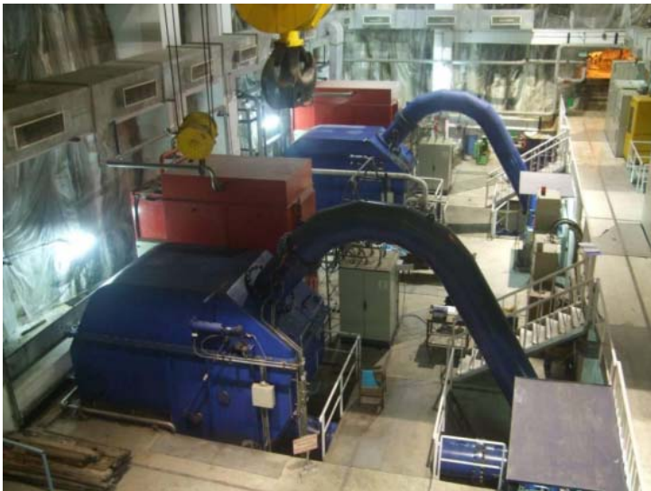
OLPD Testing of 11 kV Hydro Generators (Power Generation Customer, Nepal)
