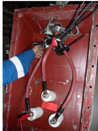
HFCT Installation in an Ex/ATEX HV motor terminal box
