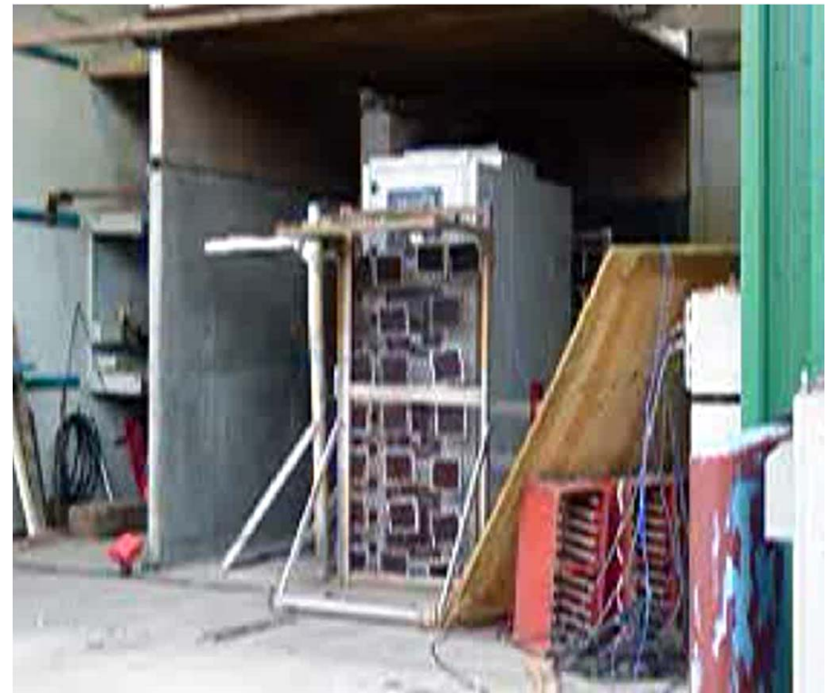
High Resistance Grounded 3 phase 80kA .5 sec
