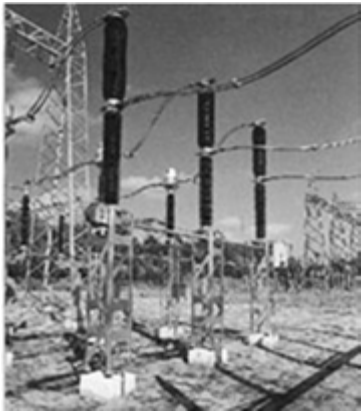
Two types of Live Tank GCB
