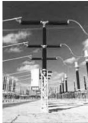
Two types of Live Tank GCB
