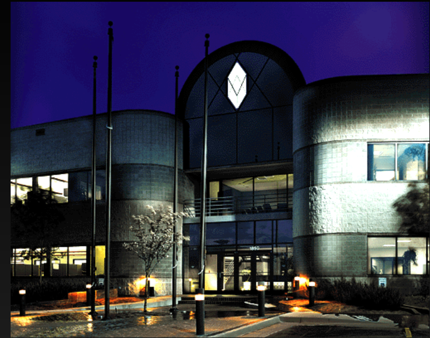
Ramtron HQ in Colorado Springs
